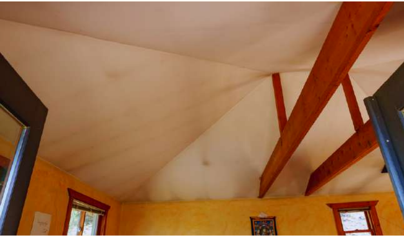
Ceiling ready to be lovingly restored
