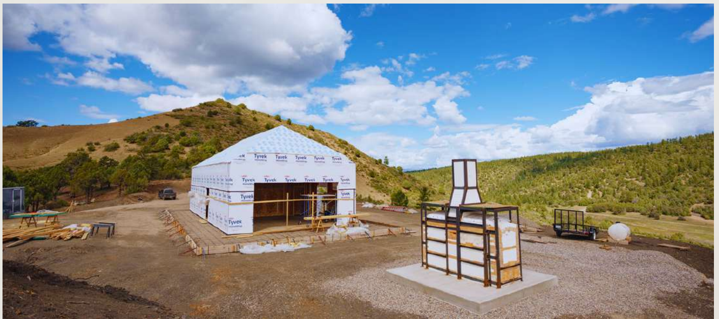
Progressing construction of the Zhitro temple at Tara's Pure Land
