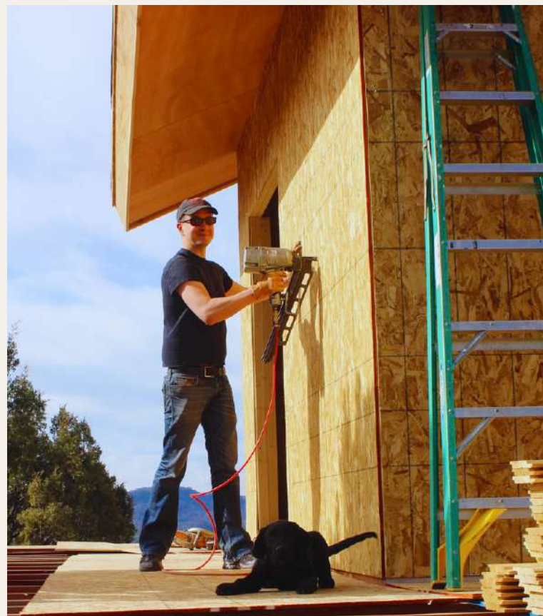
From the Archives: Cabin exterior walls installed
