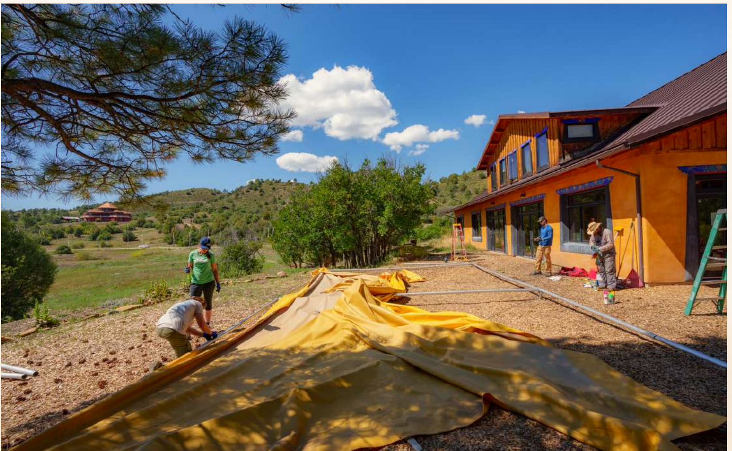
Taking down the dining tent outside the Community Building at Tara Mandala
